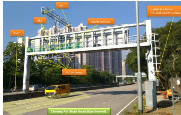
FFTS POC Study under Agreement No. CE9/2013 (HY) Tseung Kwan O – Lam Tin Tunnel - Design and Construction
